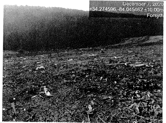
Photo Number: 4 of 4 Date: 12/7/2020 Time: 8:00 a.m. Weather: overcast Location: Greenleaf Recycling Landfill County: Forsyth Photographer: Jason Rogers Observations: Exposed litter on landfill area outside of working face.
